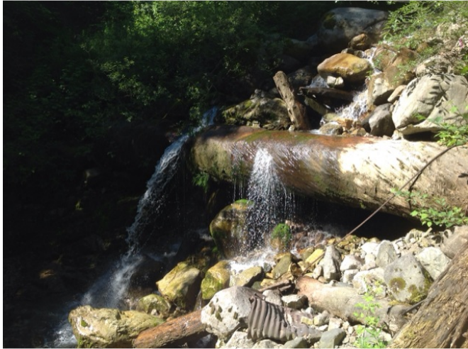
log holding back fill
