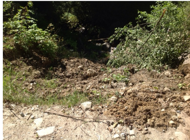
left downstream approach fills
